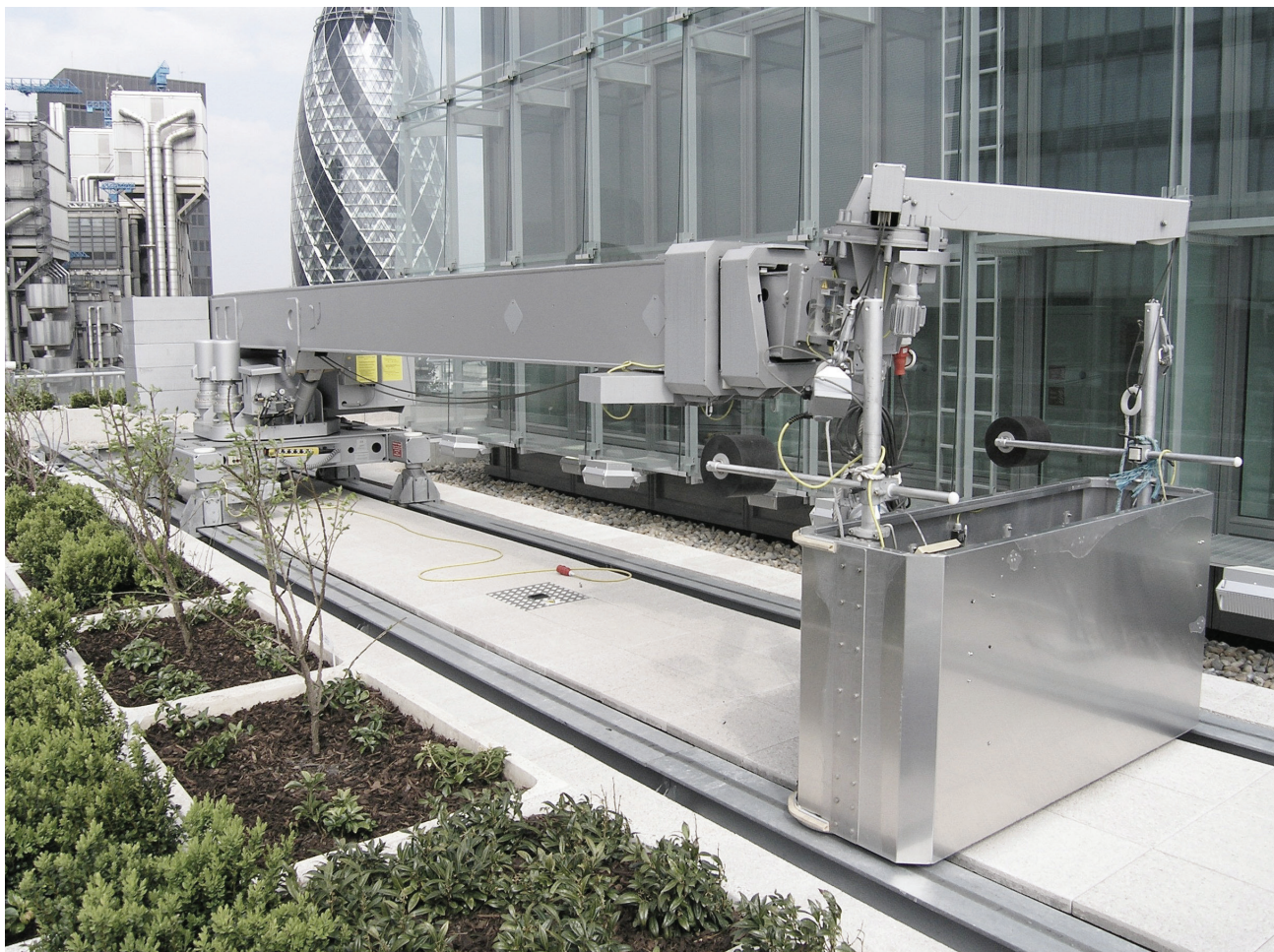
Low profile construction with double telescopic jib, track system integrated in green roof system
