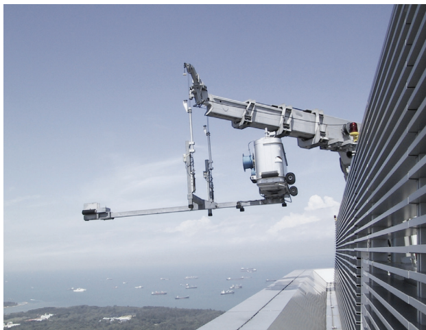
Lowering device, 3 stage telescopic jib and satellite cradle for reaching recesses in building
