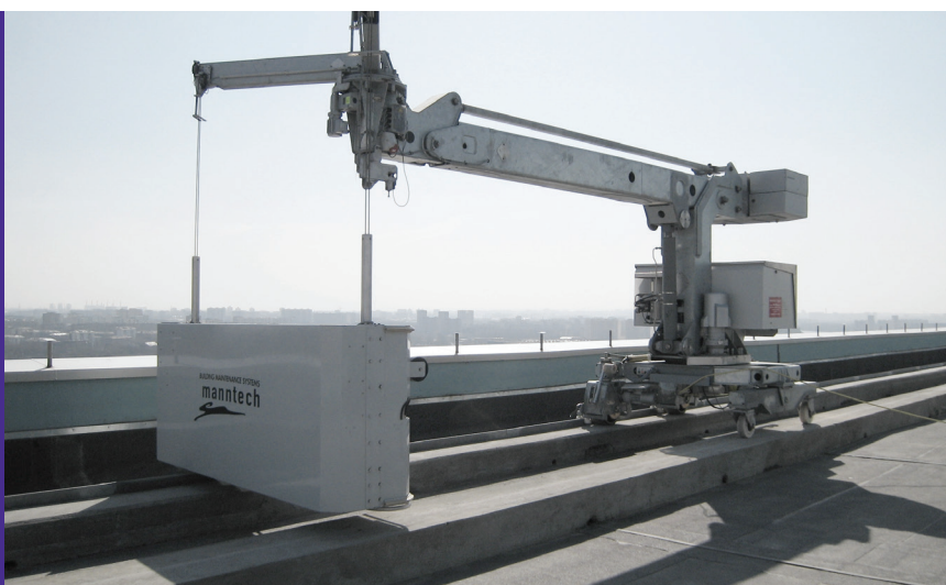
Luffing jib and coupling bar for slewing head alignment
