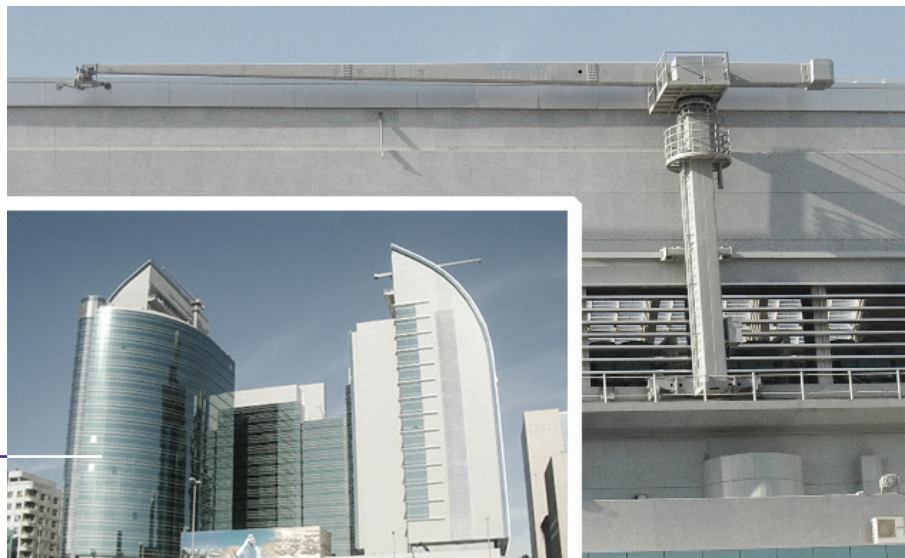
Telescopic slewing mast and maintenance platform for hidden parking position
